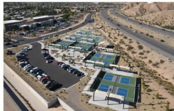
Old Mill Pickleball Complex 49 W Old Mill Rd
